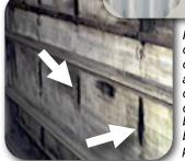
Filter Rack directly in front of coils arrows point to dirty coils caused by bypass between pleated filters.
